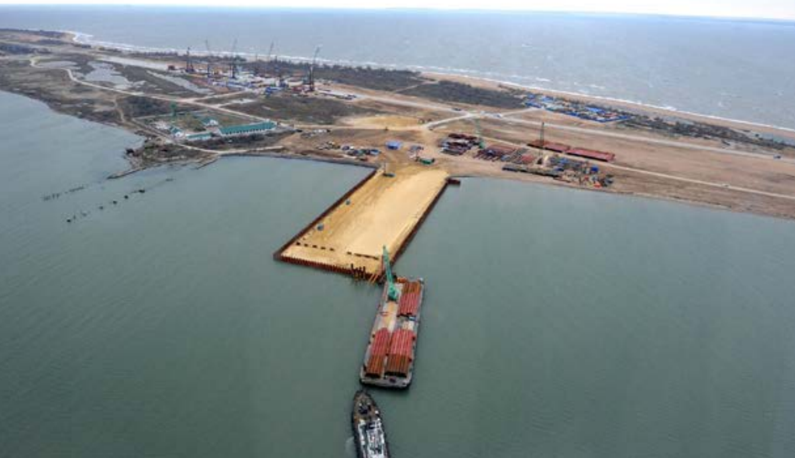
While several Ukrainian companies have initiated legal action over assets seized in Crimea, Russian authorities have proceeded with the construction of the Kerch Strait Bridge. Photo credit: The Presidential Administration of Russia
