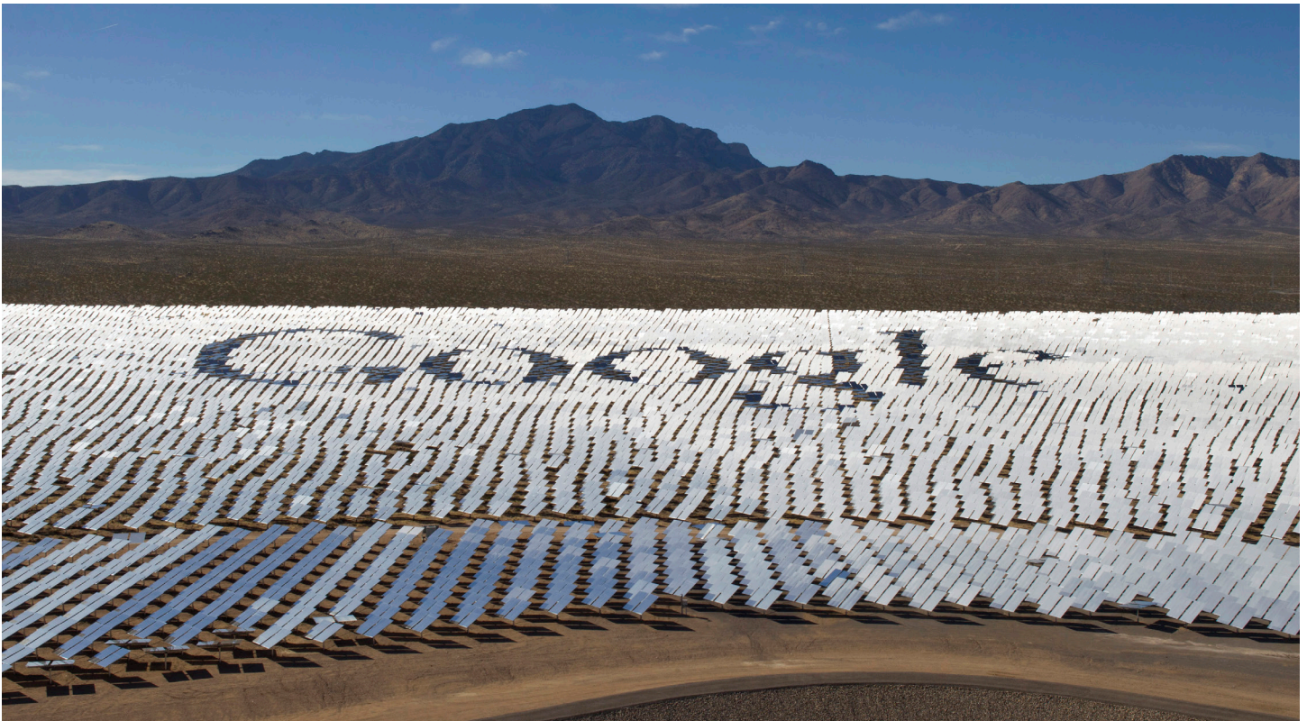
The Google logo is spelled out in heliostats (mirrors that track the sun and reflect the sunlight onto a central receiving point) during a tour of the Ivanpah Solar Electric Generating System in the Mojave Desert near the California-Nevada border February 13, 2014. The project, a partnership of NRG, BrightSource, Google and Bechtel, is the world's largest solar thermal facility and uses 347,000 sun-facing mirrors to produce 392 Megawatts of electricity, enough energy to power more than 140,000 homes. Credit: REUTERS/Steve Marcus
