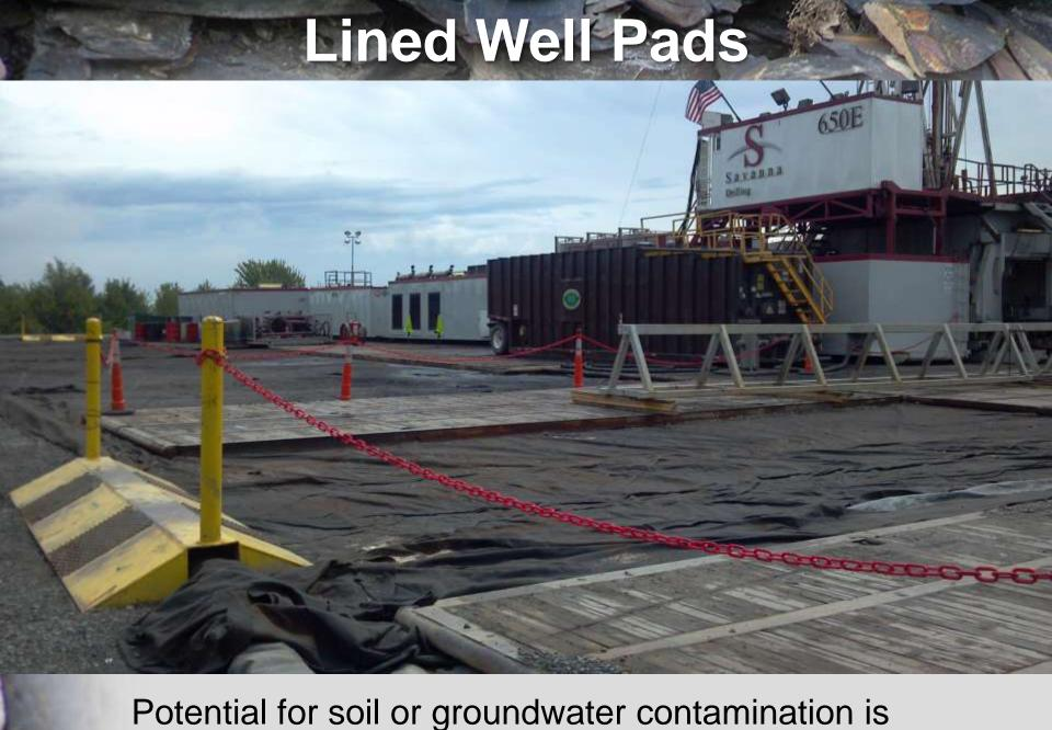
Potential for soil or groundwater contamination is minimized with lined well pads.
