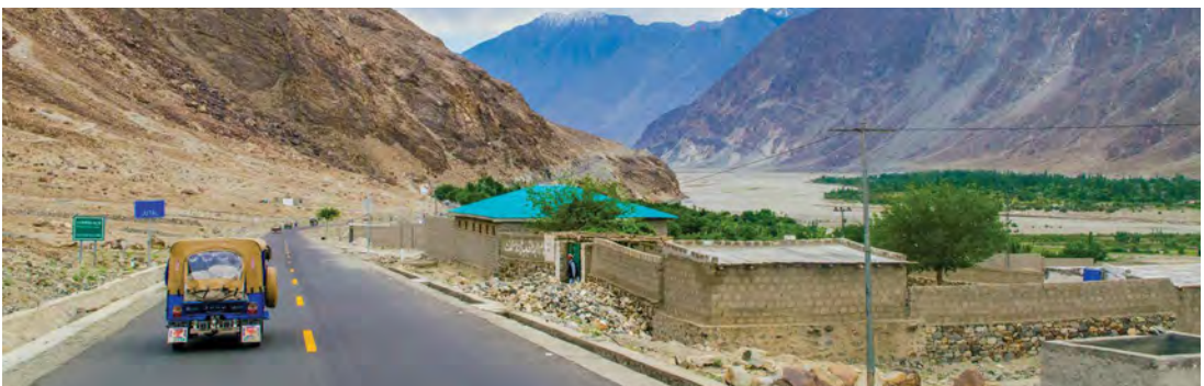
Karakoram Highway, one of the world's highest paved international roads connecting Xinjiang with the Gilgit-Baltistan region of Pakistan. Source: Wikimedia Commons.
