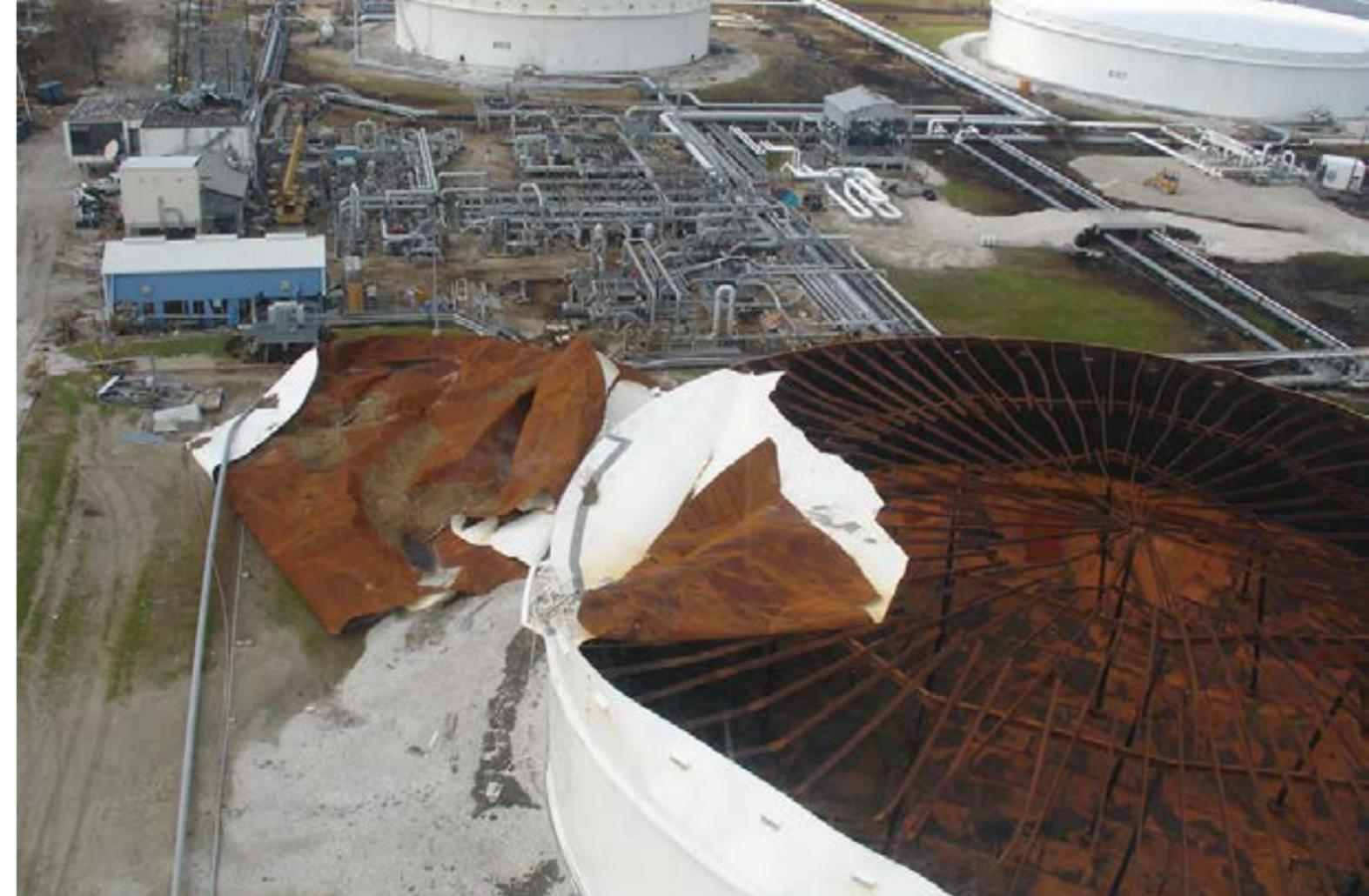
During Hurricane Katrina in 2005, one of the Chevron oil terminal's storage tanks was severely damaged on top, possibly after being hit by something extremely large carried by the storm waters. (NOAA)
