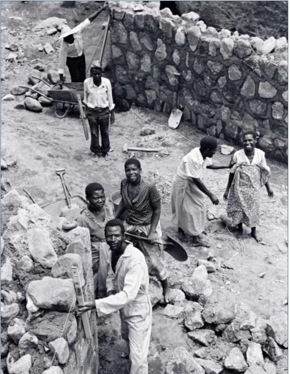
Building roads and bridges, Mozambique
