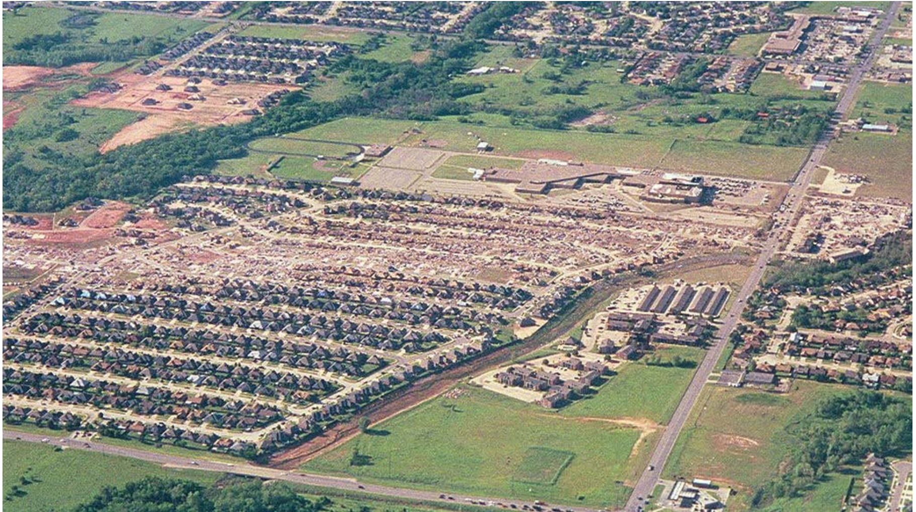
F5 damage at Moore, OK, May 1999
