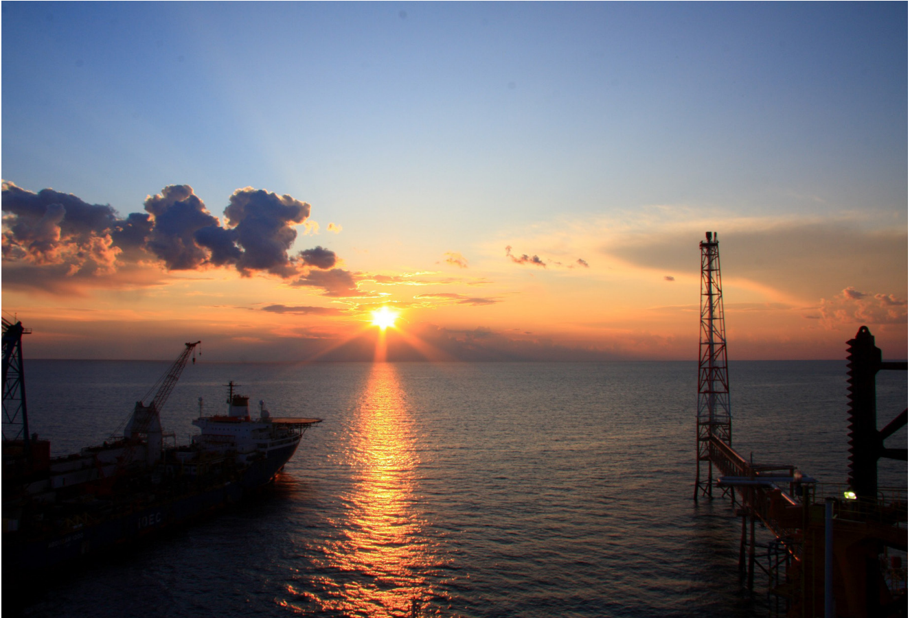
South Pars, an offshore gas field located in the Persian Gulf, is set to play a central role in Iran's energy future. Photo credit: Alireza824/Wikimedia Commons.
