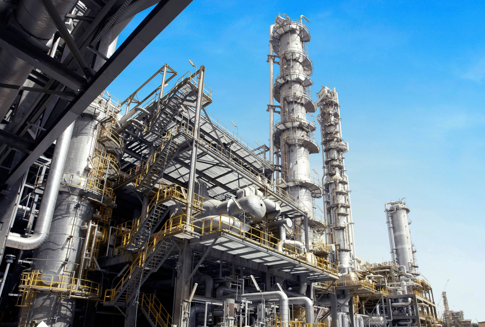
Tasnee Petrochemical Plant in Saudi Arabia. Photo credit: Secl/Wikimedia.
