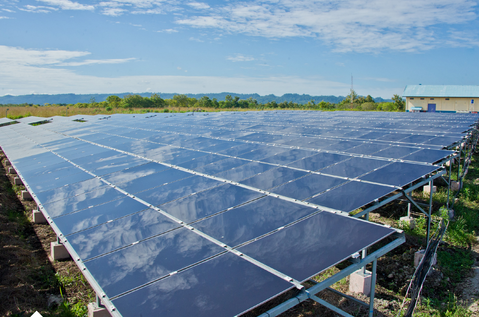
Solar panels installed to provide electricity in Sumba Island, Indonesia. Photo credit: Asian Development Bank/Flickr.
