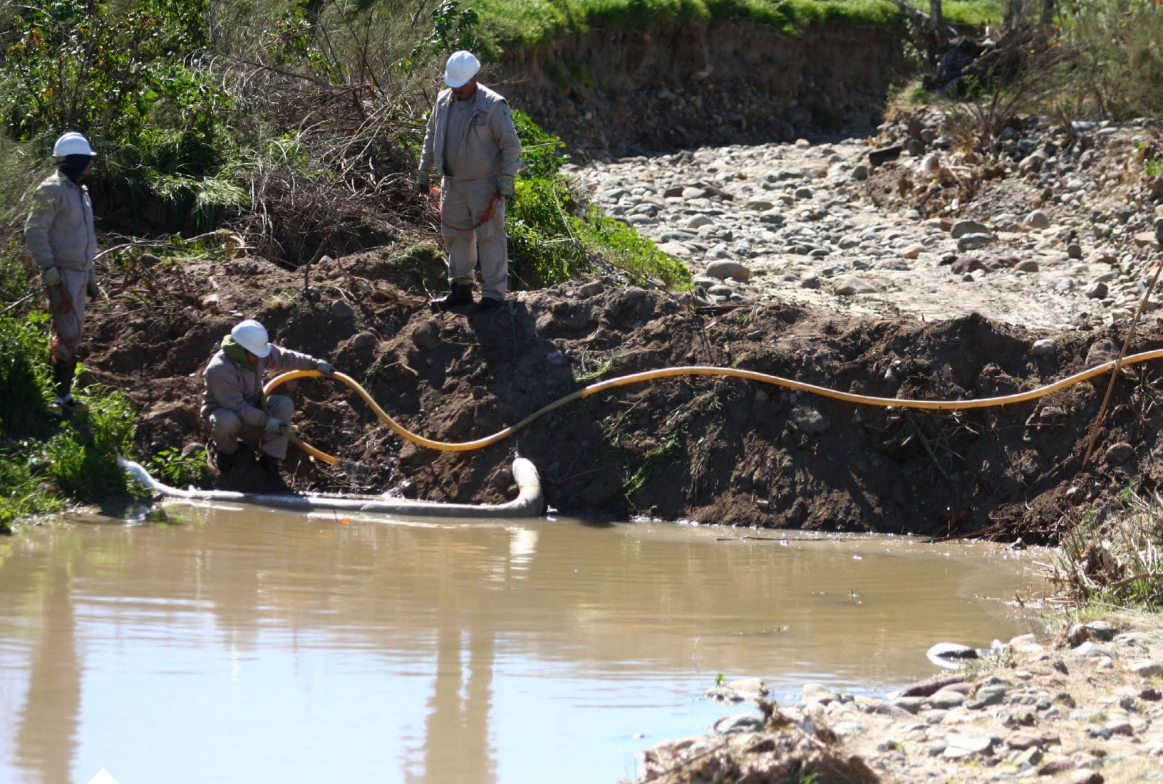
Workers from the state-owned oil company Pemex work around an oil spill near Rosarito February 10, 2011. Thieves tapping into a Mexican fuel pipeline triggered a large diesel fuel spill south of the border city of Tijuana, Mexico. Photo credit: Reuters/Jorge Duenes.
