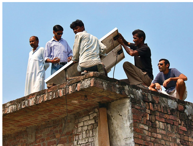
Mera Gao Power (MGP) designed a solar-powered, village-level microgrid to provide electricity to off-grid villages in India. Through the microgrid model, renewable power is generated by solar panels and stored in battery banks that charge during the day and are discharged at night. DIV provided Stage 2 funding for MGP to establish its first commercial microgrids. Flickr/DIVatUSAID (US Agency for International Development's Development Innovation Ventures program)
