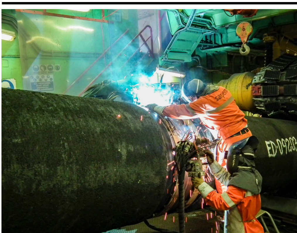
WELDERS WORK ON THE CASTORO SEI PIPELAYING VESSEL. WIKIMEDIA COMMONS/BAIR175
