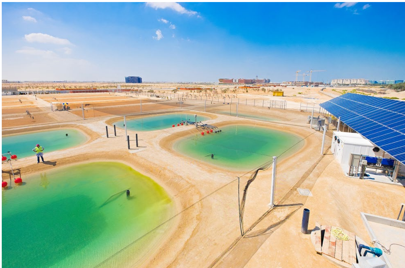
The Masdar Institute Seawater Energy and Agricultural System (SEAS) is a pilot research facility that will evaluate a process to grow seafood and biomass for food, fuel, and byproduct production using seawater. Credit: Sustainable Bioenergy Research Consortium
