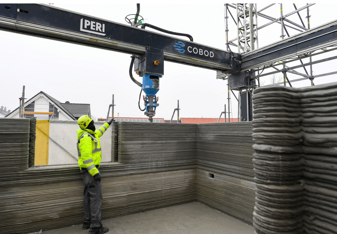
The wall of an apartment house is being printed by a 3D printer in Wallenhausen, Germany, November 25, 2020.
