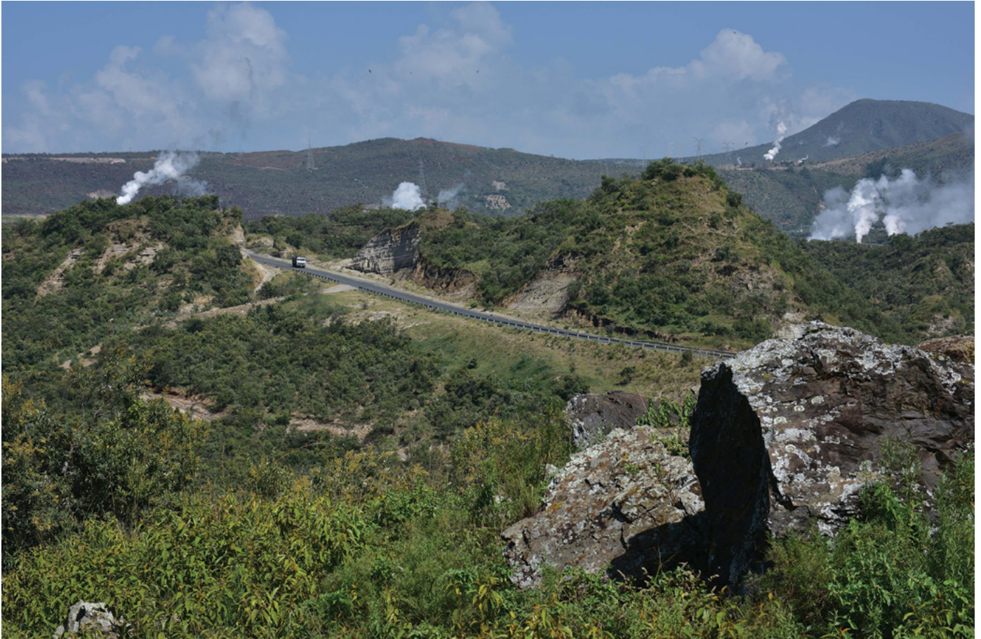
Geothermal power plants spot the landscape of Hell's Gate National Park in Kenya. Photo credit: Flickr/orientalizing. ( https://creativecommons.org/licenses/by-nc/2.0/ )
