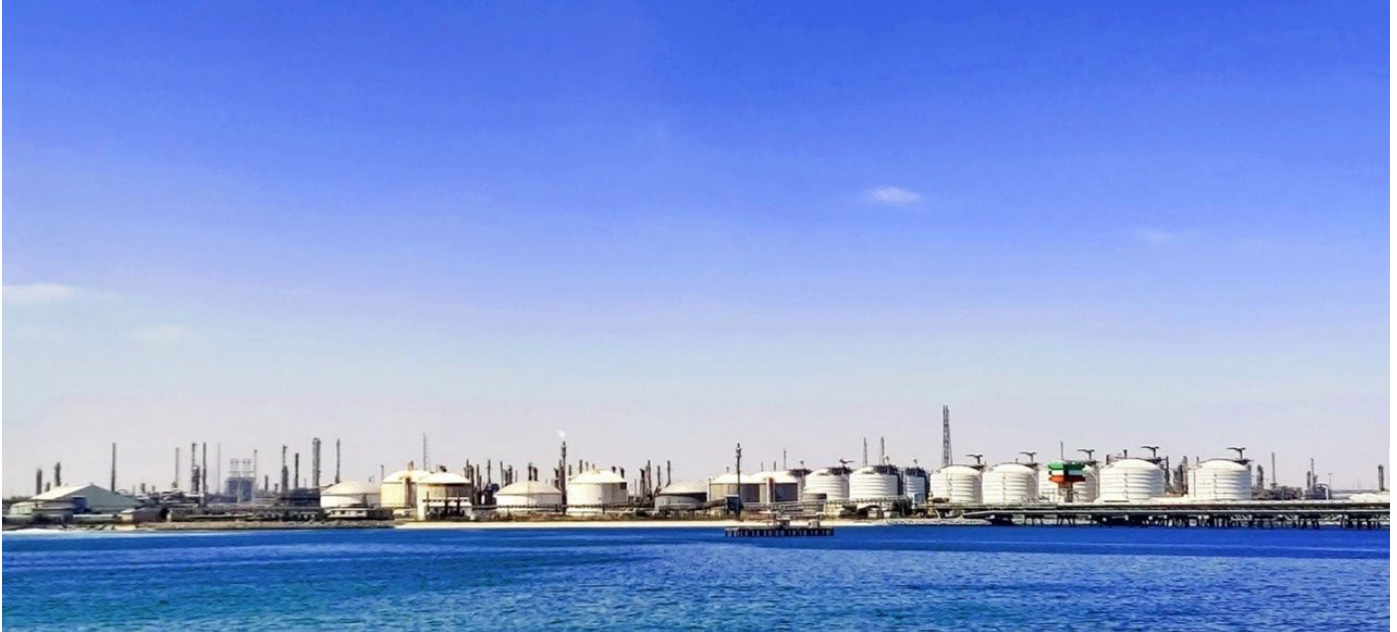
Tank farm for crude oil storage. Source: Pixabay
