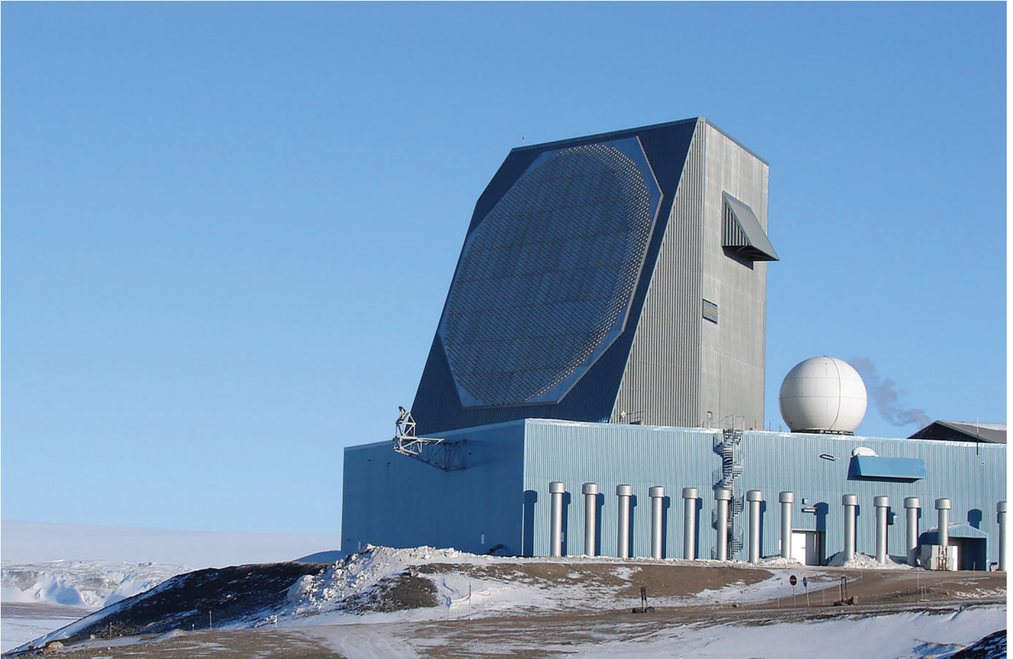
The dual-sided ballistic missile early warning radar Thule AFB, Greenland. The range of early warning radars is limited by the curvature of the Earth. Courtesy photo US Air Force.
