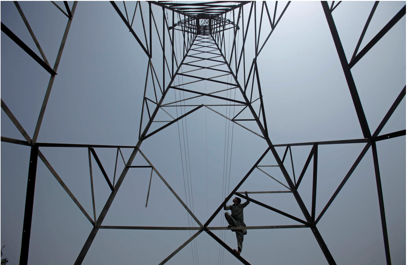
A Peshawar Electric Supply Company (PESCO) worker climbs up a high-voltage pylon in Peshawar, Pakistan. REUTERS/Fayaz Aziz
