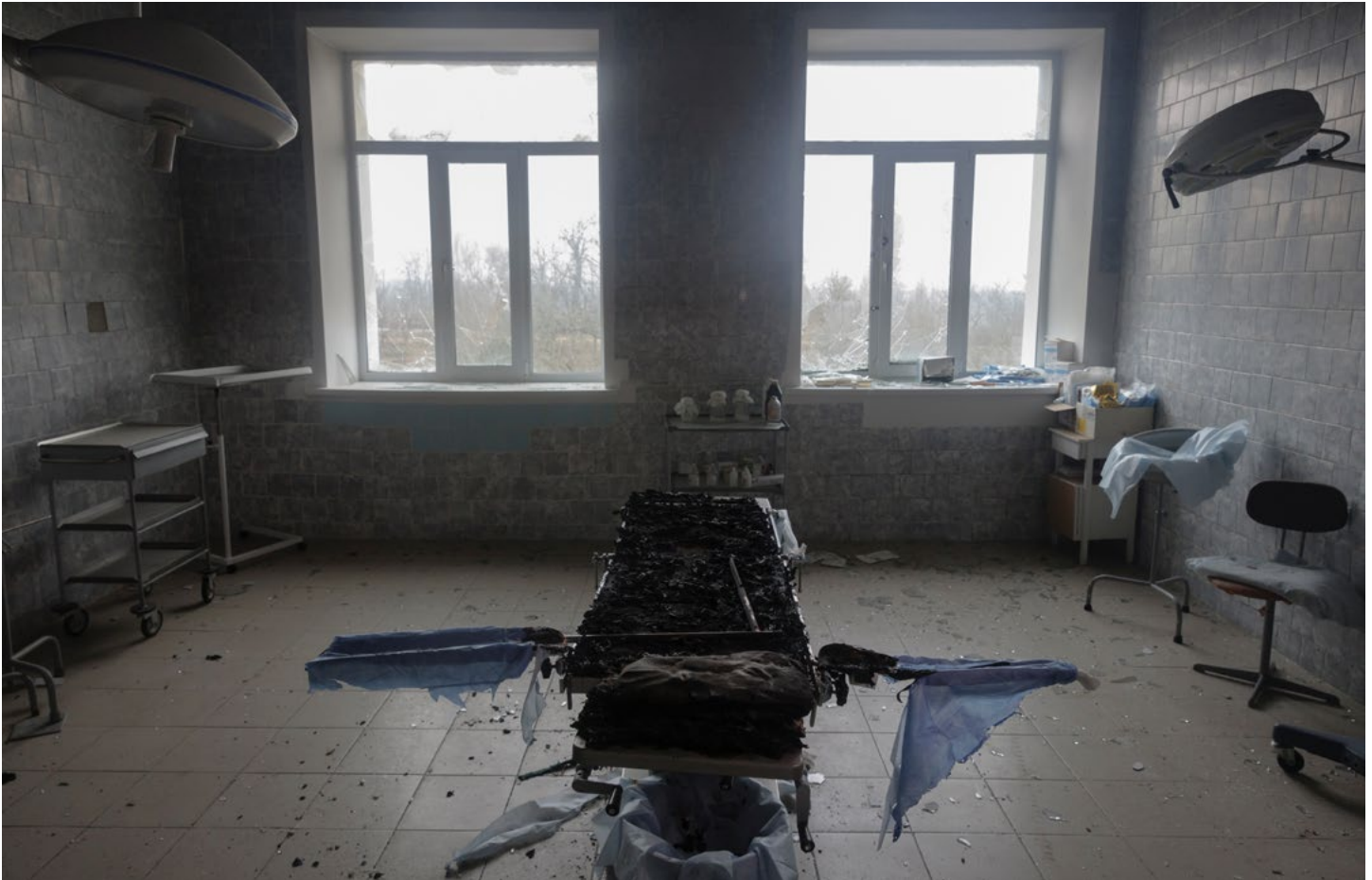
A damaged operating room in a hospital in Trostyanets, Ukraine, which staff said Russian troops attacked with tanks during their occupation of the town. March 30, 2022. Source: REUTERS/Thomas Peter
