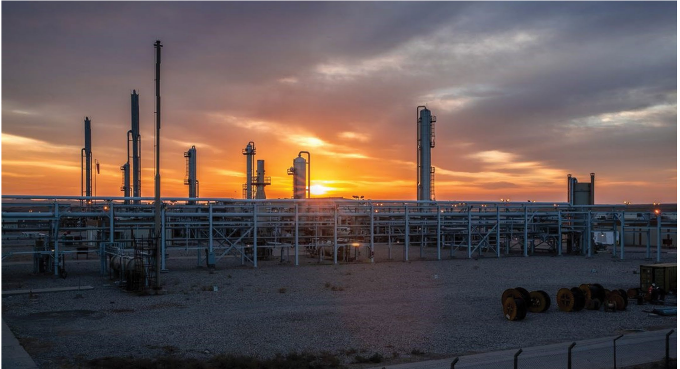
Khor Mor Gas Plant Infrastructure. Source: Crescent Petroleum.
