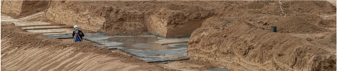
A man works at Khor Mor gas plant in Iraqi Kurdistan region. Source: Crescent Petroleum.
