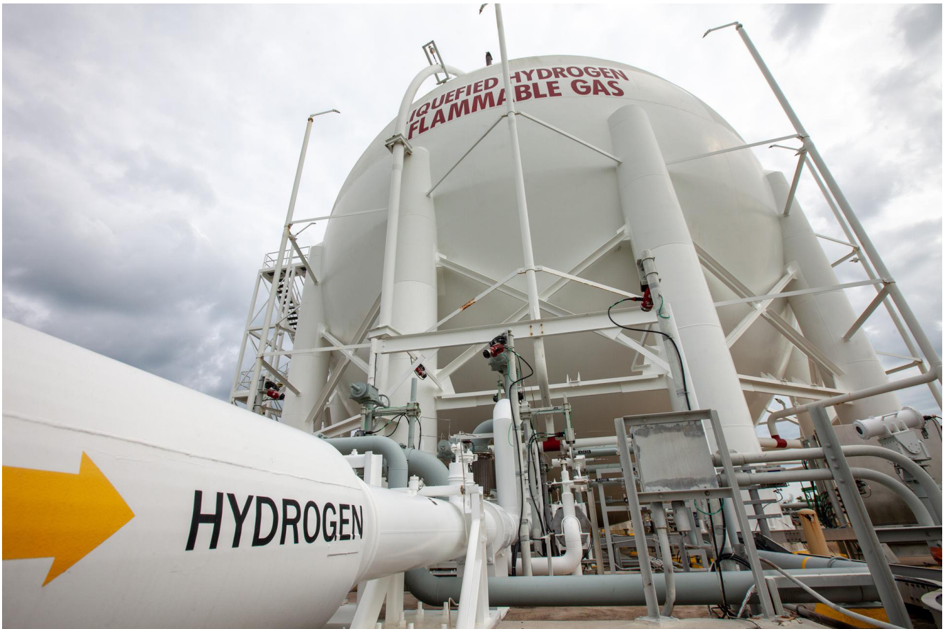
NASA's Kennedy Space Center in Florida has the world's largest liquid-hydrogen storage spheres. Much larger storage tanks will be needed to commercialize hydrogen aviation.(NASA)
