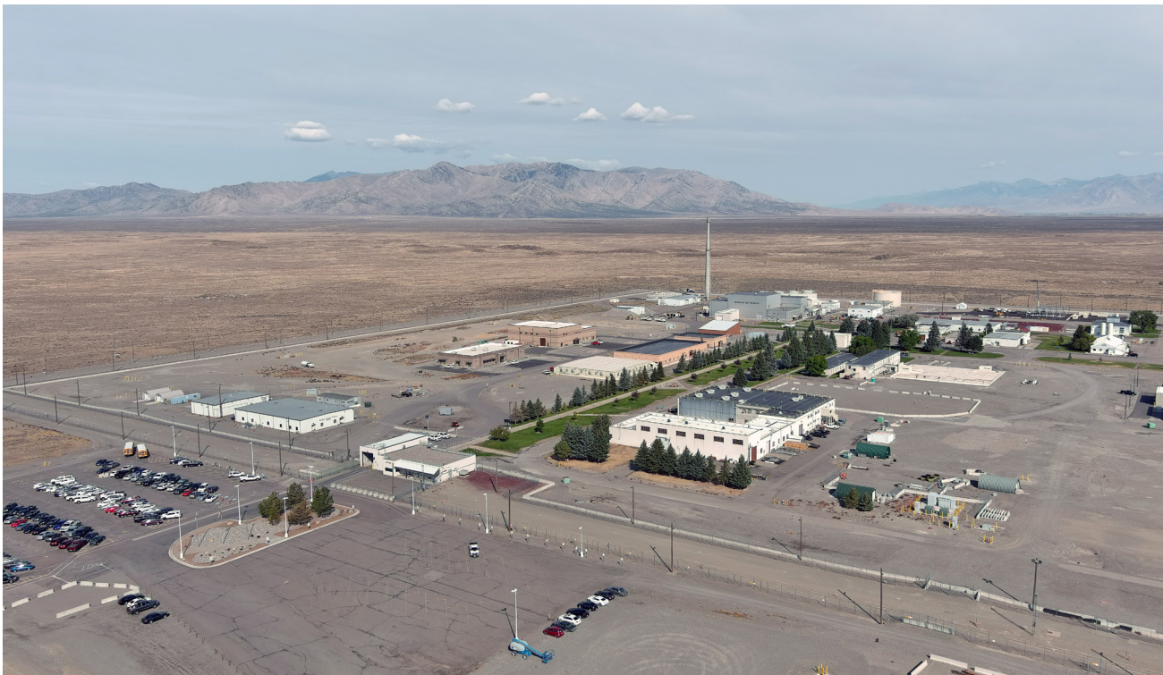
Aerial photograph of the ATR complex/reprinted with permission granted by INL.
