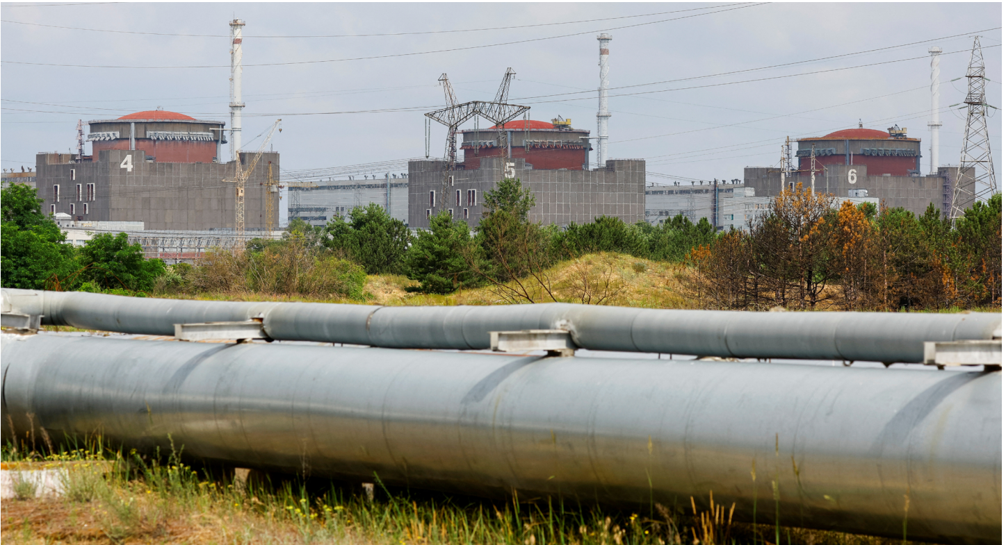
A view shows the Zaporizhzhia Nuclear Power Plant before the arrival of the International Atomic Energy Agency mission in the course of Russia-Ukraine conflict, June 15, 2023. REUTERS/Alexander Ermochenko.
