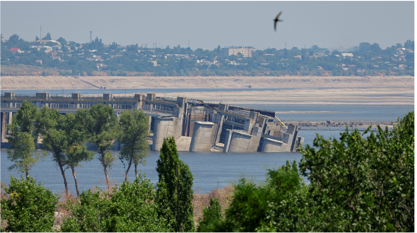
The destroyed Nova Kakhovka dam, Beryslav town and Dnipro riverbank are seen from the town of Nova Kakhovka in Kherson region, July 5, 2023. REUTERS/Alexander Ermochenko.
