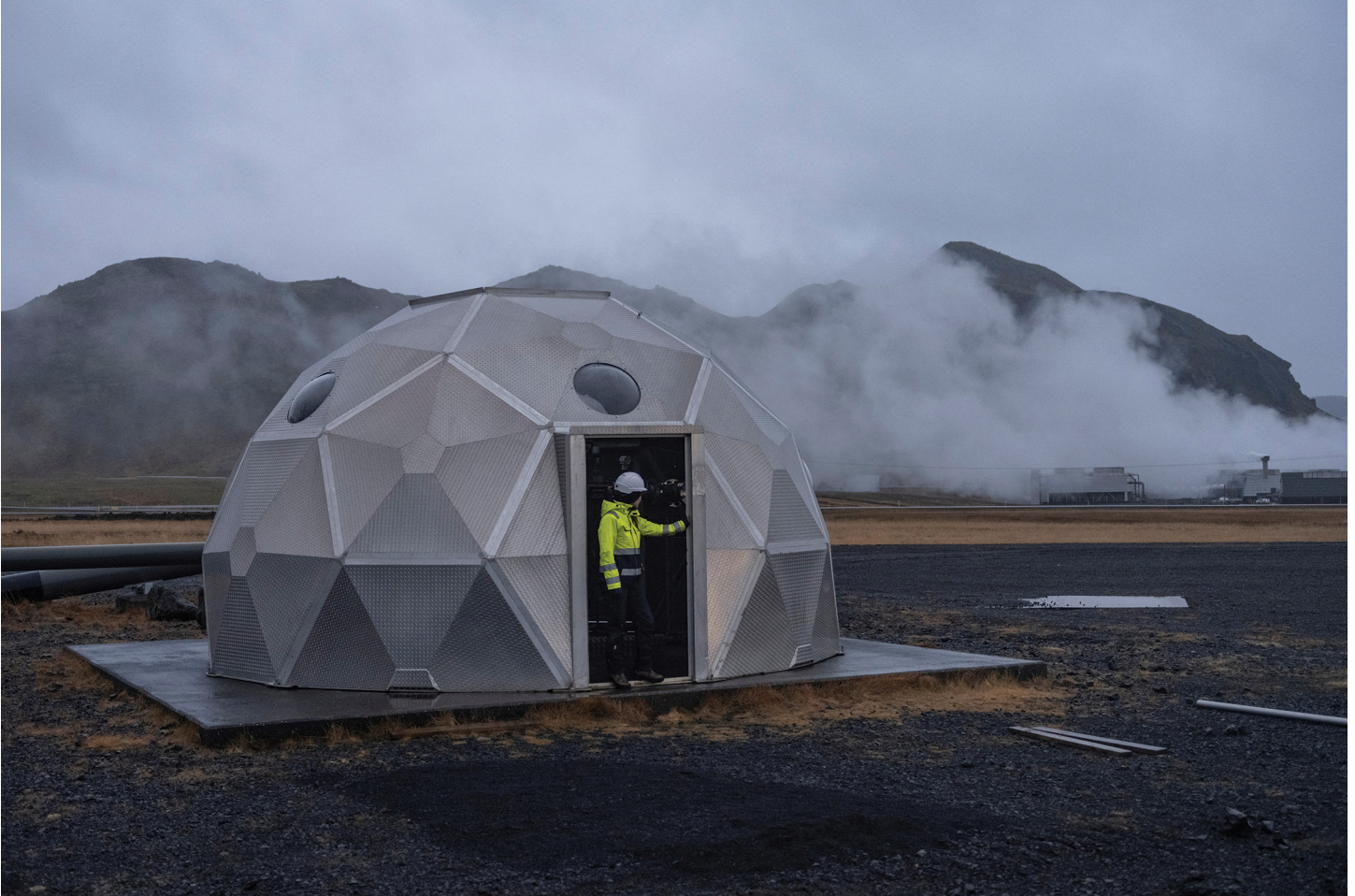
Silja Yraola, an employee of Icelandic startup Carbfix, enters the dome with injection well at its facility in Olfus, Iceland, November 21, 2023. Icelandic startup Carbfix is the world's first CO 2 mineral storage operator, permanently sequestering CO 2 by mixing it with water and injecting into basalt rock. At its facility in Olfus, on the southwestern coast of Iceland, CO 2 piped in from the nearby power plant is being mixed with water drawn up from the ground and injected into the basalt rock below. REUTERS/Marko Djurica TPX IMAGES OF THE DAY
