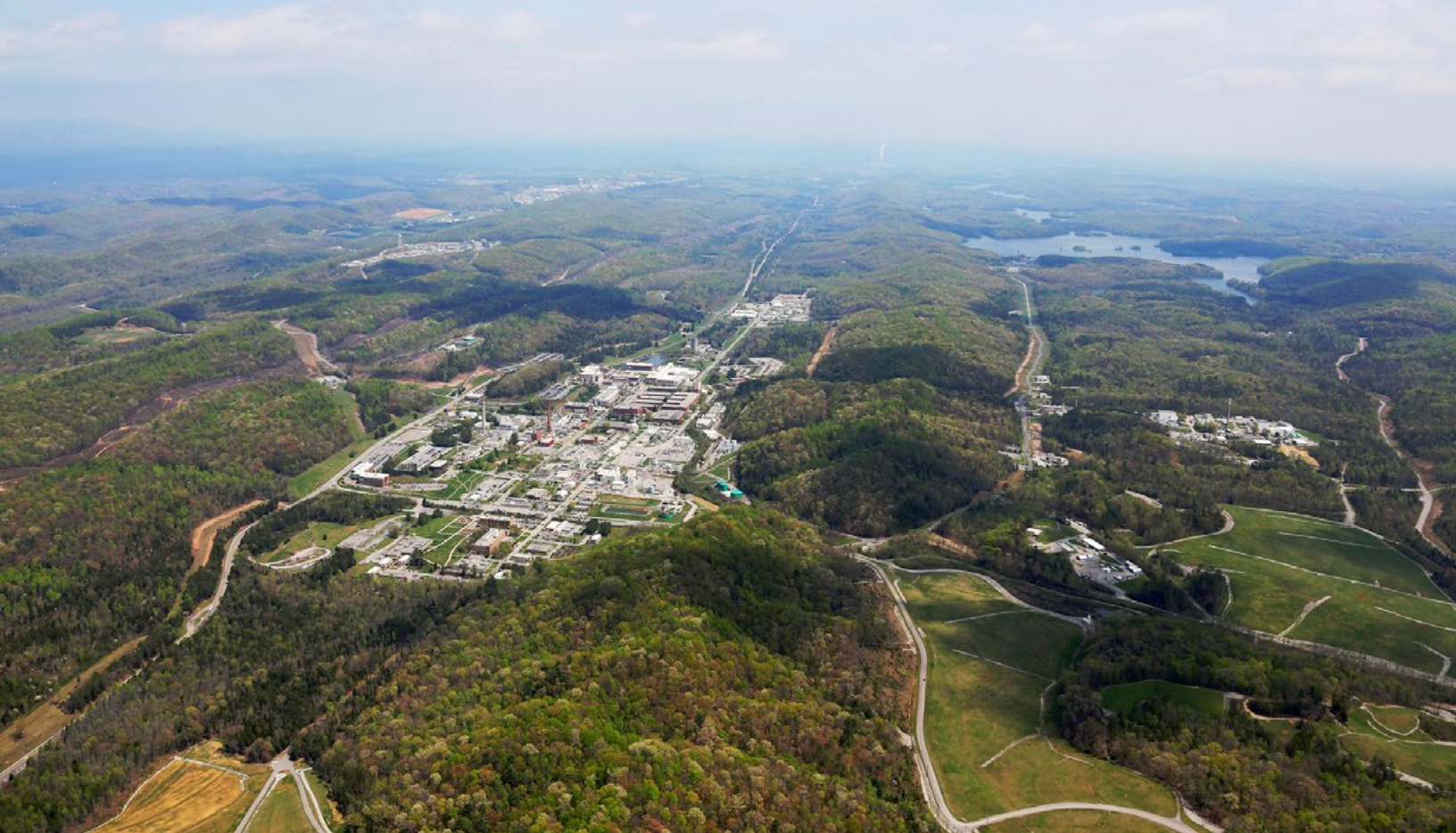
Oak Ridge National Laboratory advances the frontiers of nuclear science. Source: US Department of Energy/ORNL
