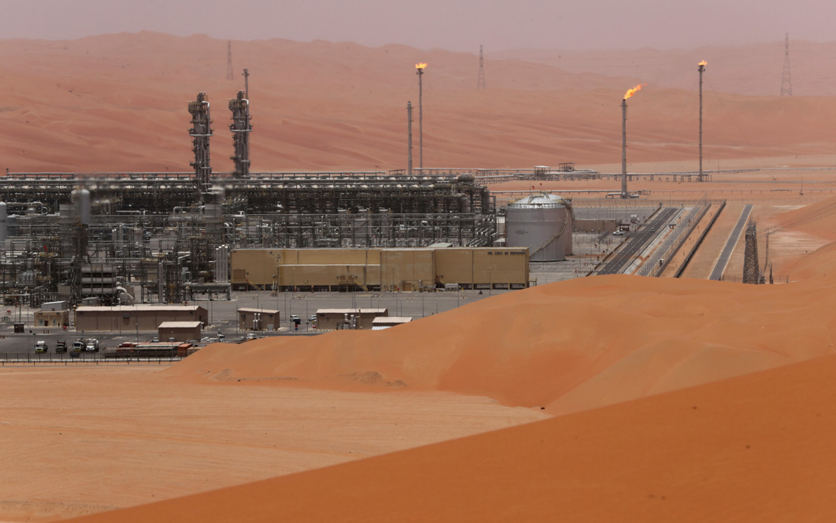
General view of the Natural Gas Liquids facility in Saudi Aramco's Shaybah oilfield at the Empty Quarter in Saudi Arabia May 22, 2018. REUTERS/Ahmed Jadallah.
