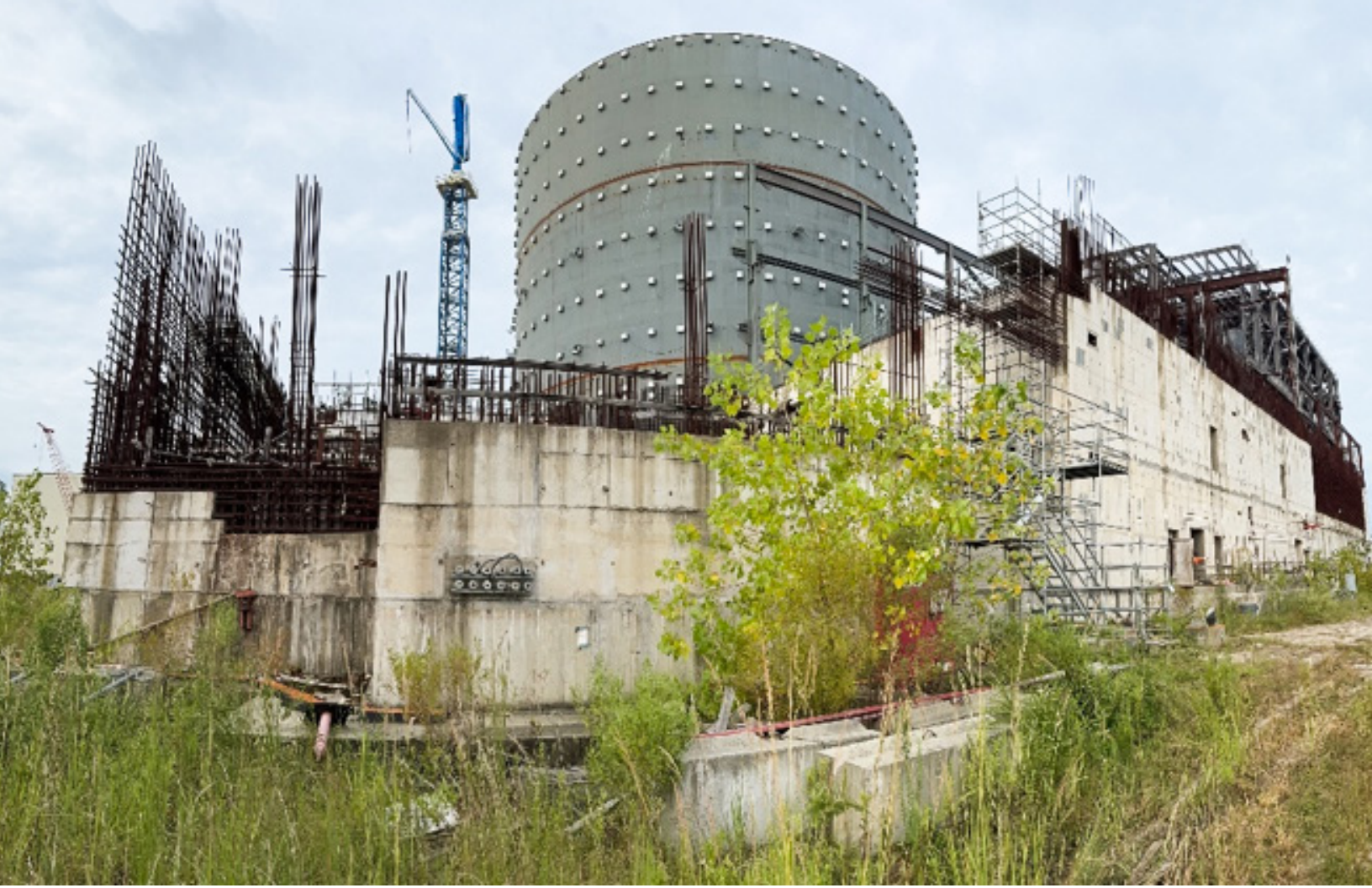
The unfinished Unit 2 reactor containment structure at the Virgil C. Summer Nuclear Plant. Source: South Caroling Nuclear Advisory Council
