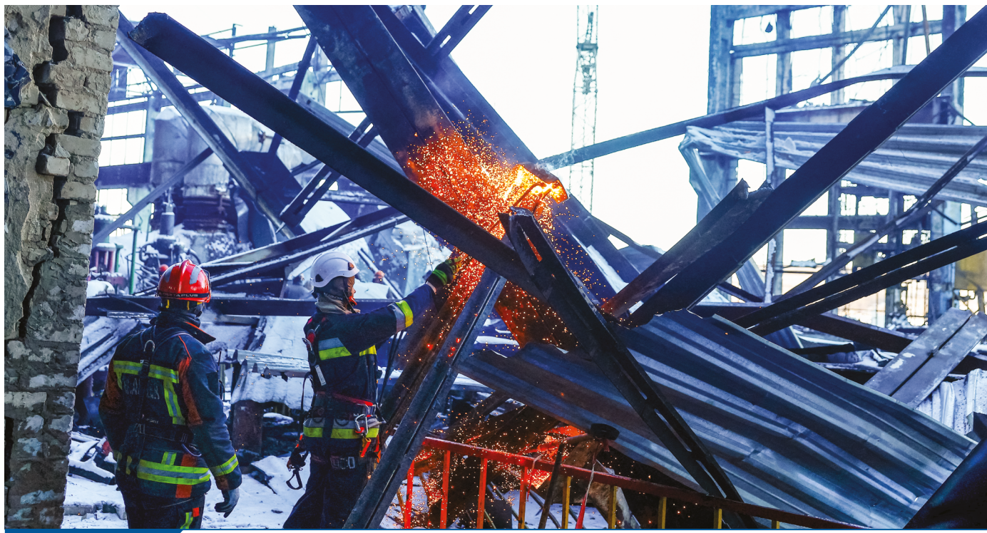
Rescuers remove debris at a thermal power plant damaged by multiple Russian missile strikes, amid Russia's attack on Ukraine, in an undisclosed location in Ukraine February 9, 2026. REUTERS/Valentyn Ogirenko
